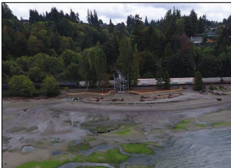
Restored shoreline at Howarth Park in the city of Everett is one of the four locations of beach nourishment along the impounded shoreline between Mukilteo and Everett. 5
