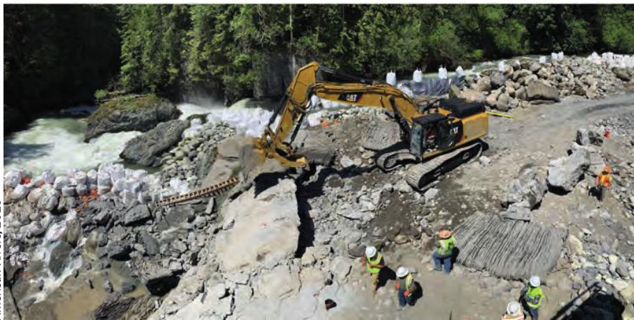
After 60 years, the Middle Fork Nooksack River Dam is being removed. 7
