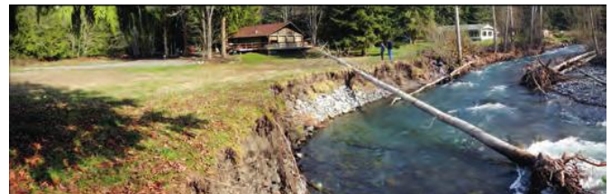
Before Restoration (March 2015)
