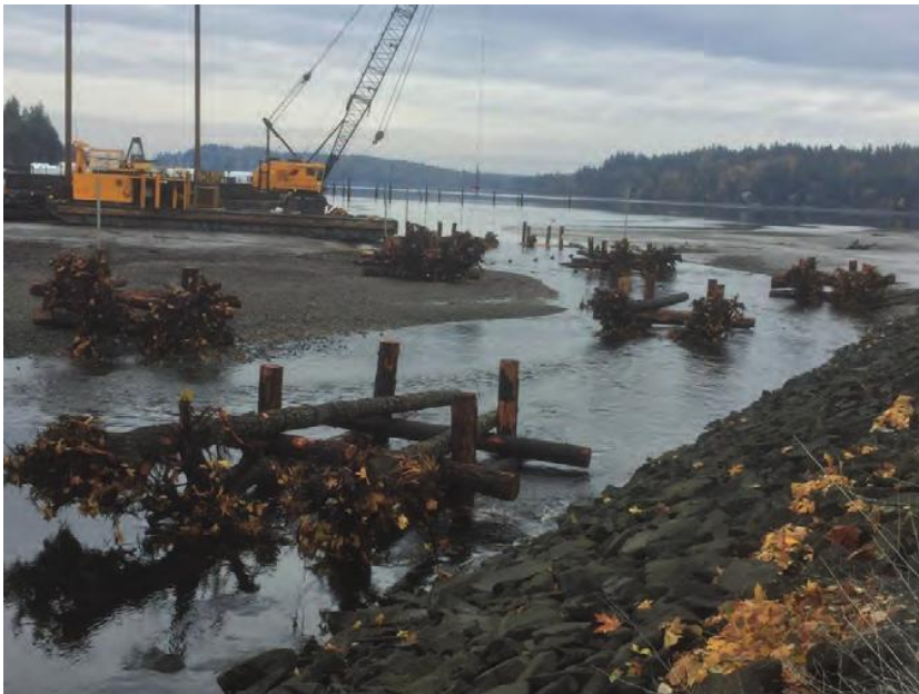
Several of the 9 logjams that were built in 2019 at the mouth of Goldsborough Creek.
