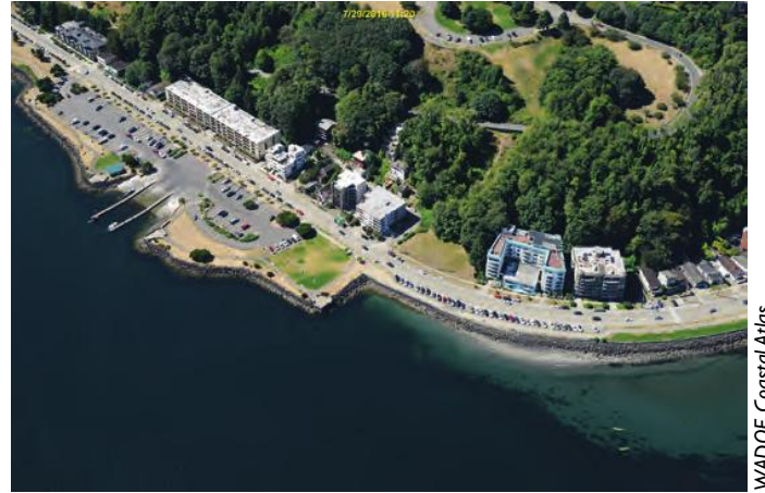
An example of shoreline armoring in King County.
