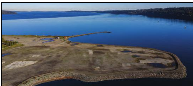
After Cleanup at Mill Site
