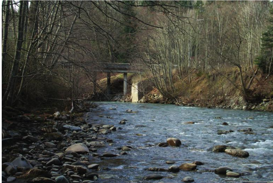
An undersized Highway 101 bridge opening on Morse Creek.
