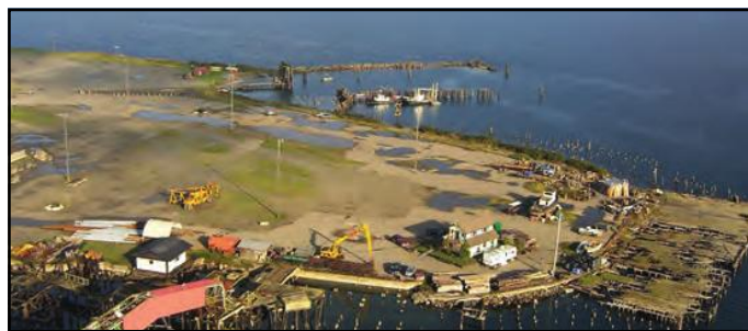
Before Cleanup at Mill Site
