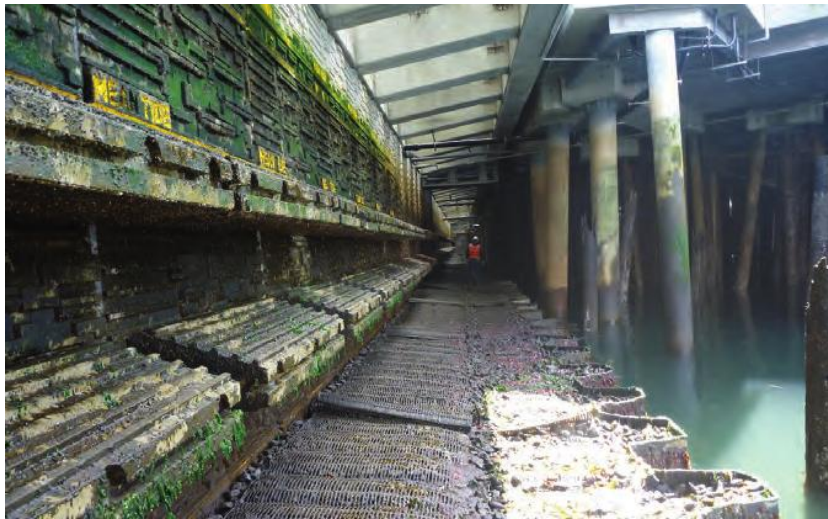
The new Seattle seawall below the sidewalk at low tide.
