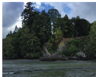
Photo 1. Bluff erosion from a 2014 slide.
