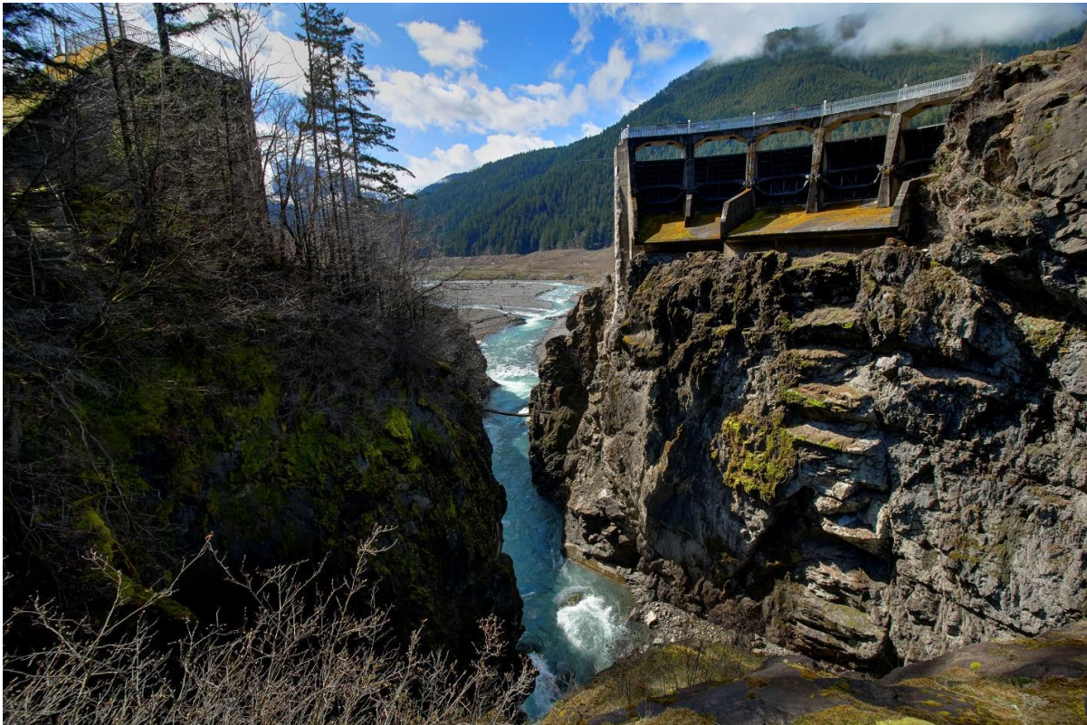
Photo: Elwha River flowing through the former site of the Glines Canyon Dam. Credit: ©John Gussman (used by agreement).
