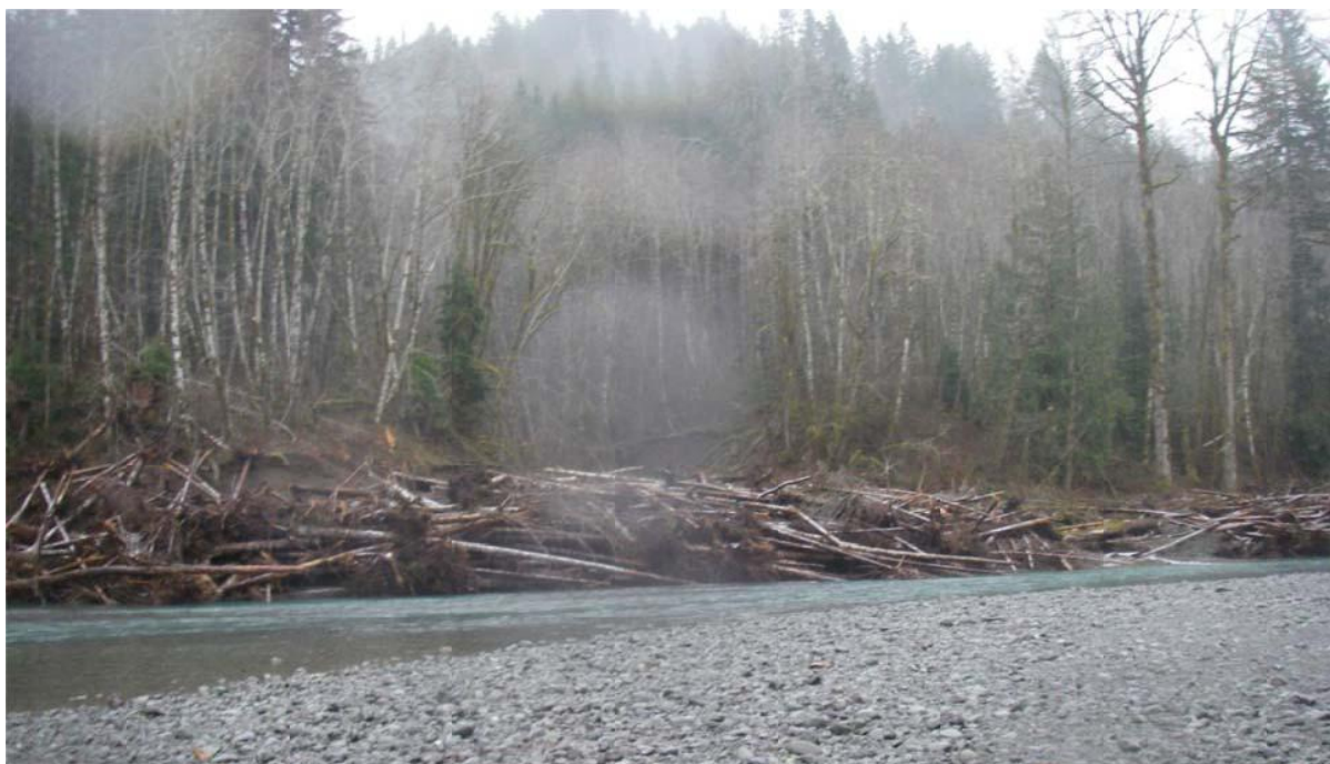
Figure 4-2. Top - Phase 1 logjam placed in the Holman Flats reach in 2010. Bottom - In November 2010, the project site experienced a major flow event. All structures that had been installed remained intact and gained wood from upstream sources.
