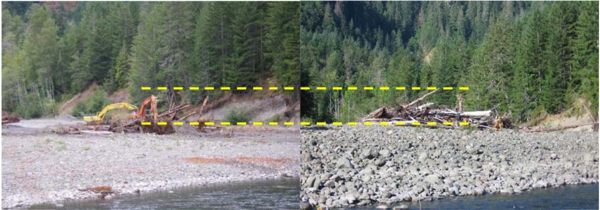
Figure 4-4. Example of changes to a gravel bar where a logjam had been built in Phase 1. On average gravel bar heights increased 2.4 feet through the project reach. Maximum accumulation height on structure #5 (shown) was 6.6 feet. From Geiger (2015).
