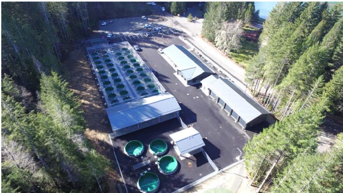
Figure 3-1. The North Fork Skokomish Hatchery built and operated by Tacoma Power under terms of the Cushman Settlement Agreement. The facility was built in 2016.
