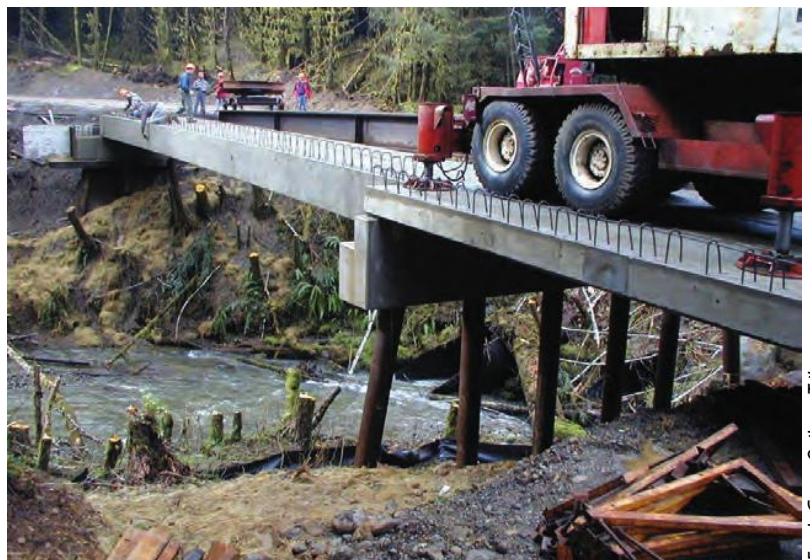
The Quileute Tribe replaced two corroded and perched culverts with a bridge in the south fork of Maxfield Creek, a lower Bogachiel River tributary.
