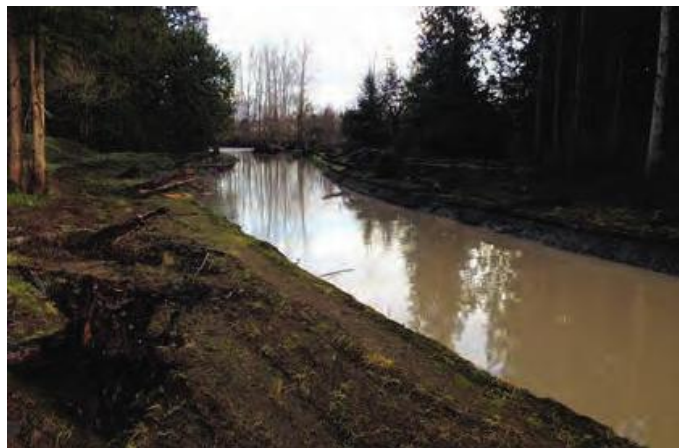
Completed South Fork Phase I Channel.
