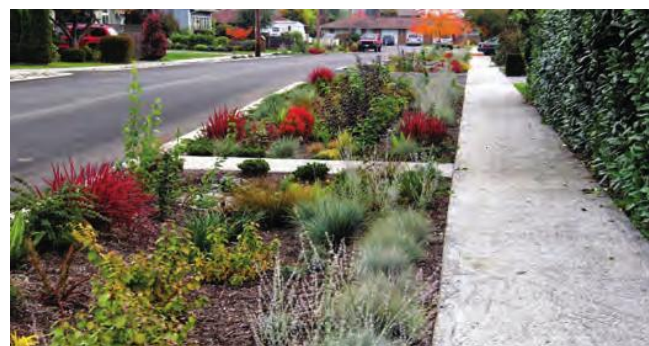
8th Ave NW Rain Gardens along the Street of Green: A rain garden is a planted area designed to filter rain water that flows from compacted or impervious areas. Rain gardens do not retain water; they only temporarily collect the water and drain within 12-48 hours. 6
