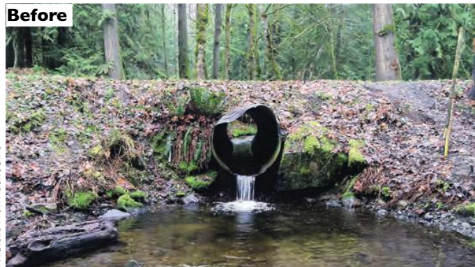
WF Clear Creek Culvert Removal: To improve fish passage and enhance habitat, Kitsap County permanently closed Sunde Road at Clear Creek and removed the culvert in the summer of 2013. In addition to improving fish passage, this project restored instream and riparian habitat and improved water quality.
