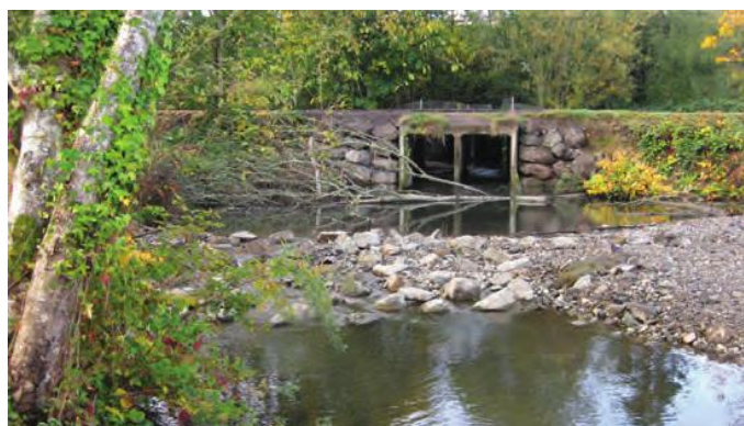
Kittyhawk Drive and culvert at mouth of Chico Creek, prior to removal of the road/culvert and restoration of the estuary.
