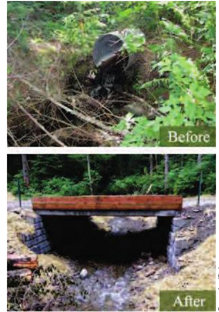
Example of RMAP road and culvert repair.
