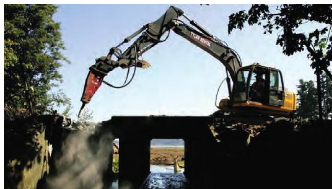
Workers pulverize Kittyhawk culvert.
