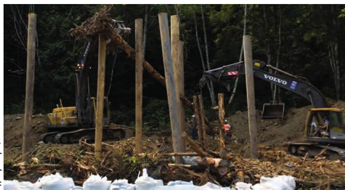
Logjam installation on Morse Creek
