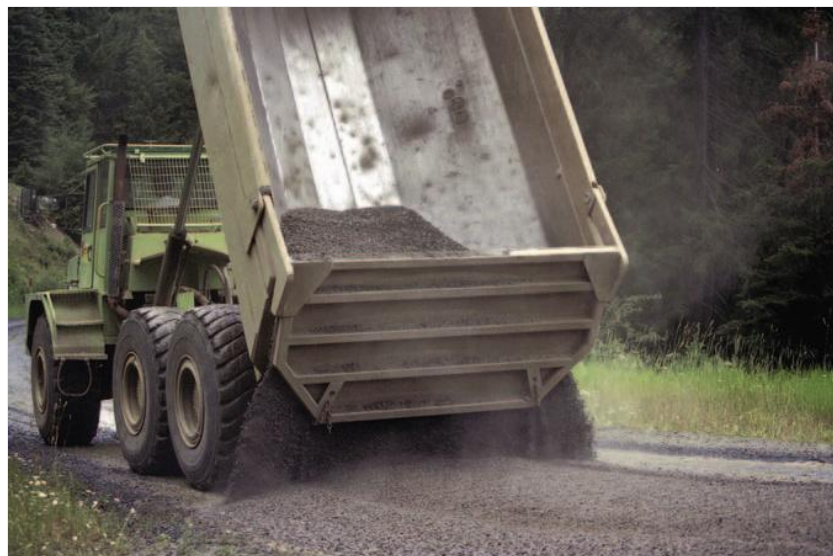
Roads on working forestlands are being repaired and maintained to prevent sediment from entering streams. Photo by Keith W. Wood, courtesy the Washington Forest Protection Association.
