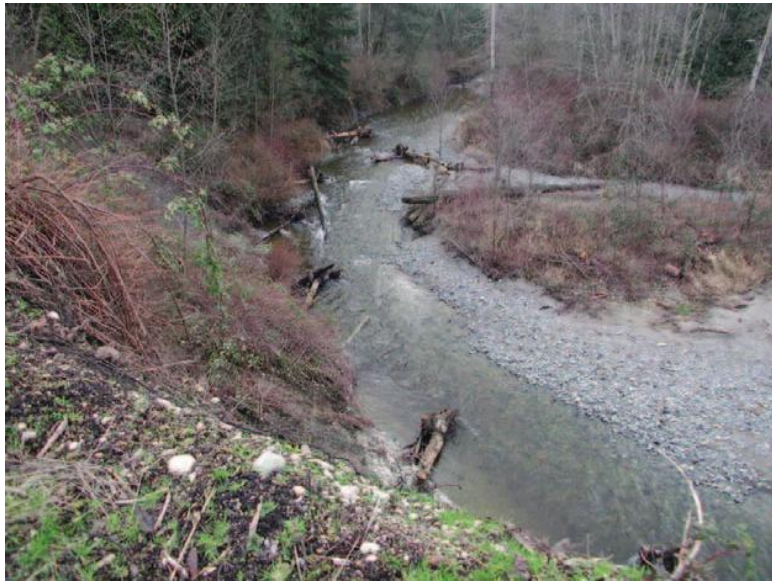
Photo courtesy the Washington State Salmon Recovery Funding Board
